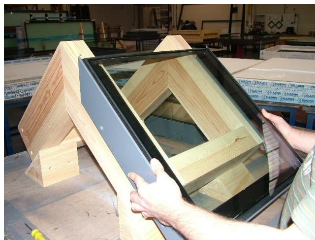
Figure 8 – Installing the first half of the unit
