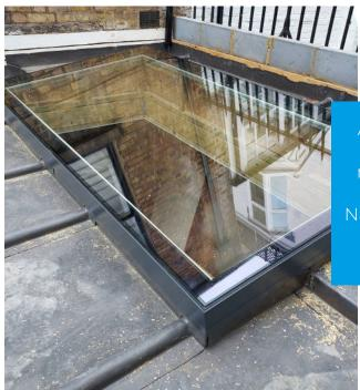
Accessing the garden flat posed a challenge due to its unique layout. The most difficult task was manoeuvring the glass components required for the installation of the Flushglaze Rooflight. Navigating these substantial glass panels through the challenging access points presented a considerable obstacle.
