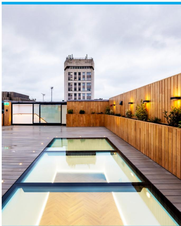
On this particular project, the sliding section when open provides a clear opening of 1927mm on the left side when viewed from the outside and is glazed on the front and top with a built-in fall of 3 degrees, and mounted to walls at the rear and two sides. The rooflight also includes the optional extras of a proximity detector and a battery back up. The rooflight was crane lifted to the terrace so that installation could be carried out by our sister company, Glazing Renovations.
