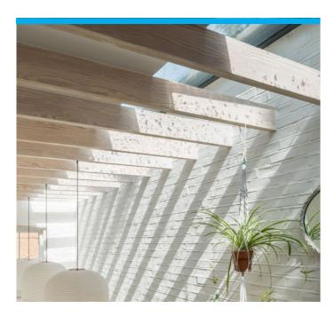
As stated, the rooflight was supplied in three sections with the frameless silicone joints segmenting each section; the three sections were sized to achieve an equal split when viewed from underneath. This meant that the end sections had to be larger to account for the upstand width.
