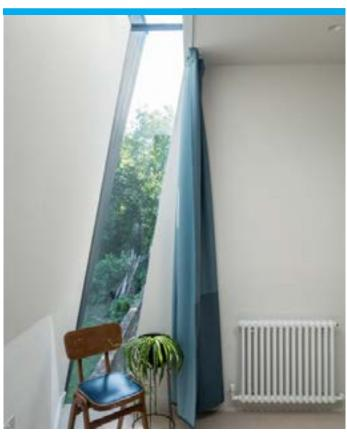
Mr Cannon and Gruff Architects decided to use the Fixed Eaves Rooflight for the soon to be family home. The Glazing Vision Eaves Flushglaze Rooflight comprises of two or more glazed sections - installed in both vertical and horizontal planes and joined together with a structural silicone seal.
