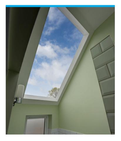
The Pitchglaze unit provides a frameless internal view so that when installed, the homeowners were able to enjoy sky only views from the roof window. Something not usually found with traditional roof window products. Two portrait orientation roof windows, measuring 2000mm x 1000mm, were used in the first floor to flood the new extension with daylight and remove the previous dark dingey corners of the home.
