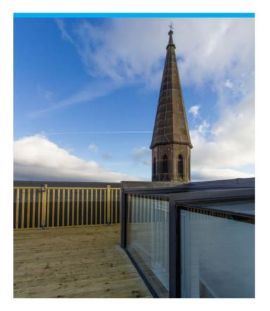
PJL needed to ensure that the building remained watertight as construction work progressed to the roof top phase. The solution was to build a new roof under the old one. Once an aperture for the box rooflight was created, the old roof was removed. This then allowed for the smooth installation of the glass box rooflight, which had been prevision-engineered to PJL's unique dimensions by Glazing Vision's dedicated team.
