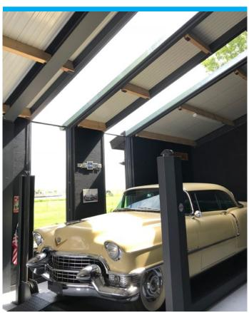
The rooflights comprise of a 2.6 metre vertical double-glazed unit, which then continues at a pitch of 18.4 degrees uninterrupted along the span of the roof for a further 4 metres. The Flushglaze units are designed to be installed completely in plane with the roof fabric, resulting in an almost frameless finish, both inside and out.
