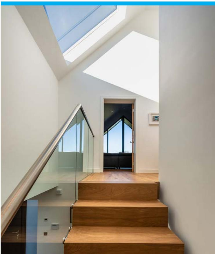
Initially, a generously sized Glazing Vision flat glass Flushglaze roof light, measuring 980mm x 2680mm, was specified to be installed over the entrance hall. This provided the clean lines and prevented any impact on the aesthetic when viewed from outside the front elevation. The frameless interval views create the perfect effect, allowing a multitude of natural daylight to shine through into the entrance hall and emphasize the impact within the home.
