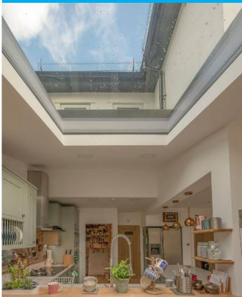
The fixed eaves rooflight, measuring 3010mm (span) x 1310mm (width) x 1556mm (height), provided a continuous view of the garden and allowed KJC Architects to focus on one tree in the garden, which they wanted to emphasise from the initial concept stage.
