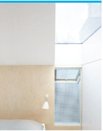
Critically Glazing Vision's Flushglaze fixed rooflights, with no visible internal framework, ensured that far from negatively impacting on the low ceiling, the room height was actually maximized and the natural light falling into the master bedroom and stairwell thereby optimized.
