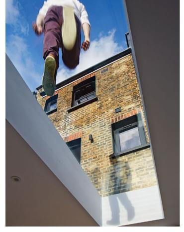
Engineered by Glazing Vision with a 25.5mm clear laminate outer pane, 14mm Argon filled warm edge spacer cavity, and 6mm heat soak tested toughened inner pane, the walk on rooflight is designed to meet the future projected foot traffic upon them with uniform loadings of 1.5kN/m² and concentrated loadings of 2.0kN in accordance with BS EN 1991-1-1-1:2002.
