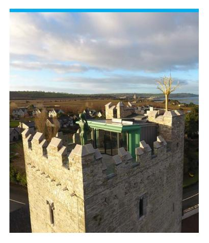
Alongside the Sliding over Roof rooflight, was a minimalistic fixed Flushglaze rooflight which provided a view from the inside of the sky and also the roof mounted sculptures. Andrew Burningham of architecture:ab explains that "externally, the minimal form of the rooflights, reduced the visual impact from long distance views of the castle".
