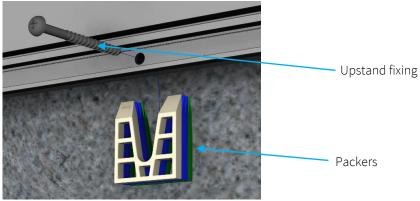
Figure 9 - Upstand fixings
