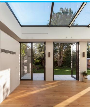
With such a complex rooflight, with fixed and sliding sections, a quiet and efficient operation was fundamental to the specification. Electronically controlled at the touch of a button, each of the 2 sliding sections of glazing can be retracted easily, revealing generous openings, and sky-only views. An added safety feature is the manual override should the electronic control system stall.
