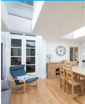
Glazing Vision were able to specify two flat Flushgaze rooflights, and a wall abutted bespoke rooflight. This allowed the homeowners to benefit from natural daylight throughout the entirety of the extension and helped to flow through the rest of the property.
