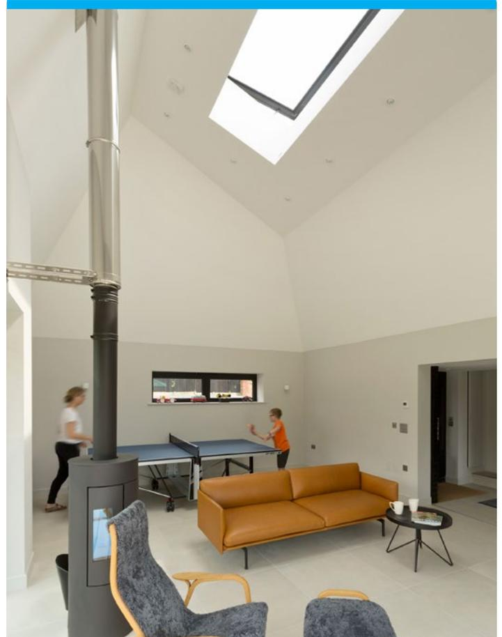
Additionally, the VisionVent rooflight provided excellent thermal performance, with the combination of 8.8mm low emissivity glass, 6mm heat soaked tested toughed glass, argon-filled cavities and 18mm warm edge spacer bars. Preventing the risk of condensation forming and ensuring that when closed, heat is retained inside the barn.
