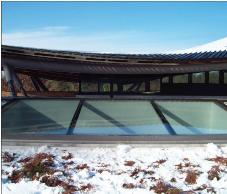
Figure 4 Typical Flushglaze installations
